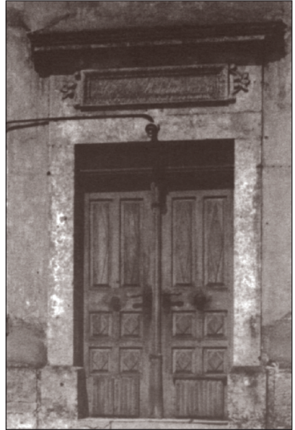
Rabensteiner Straße 1, Detail Tür
